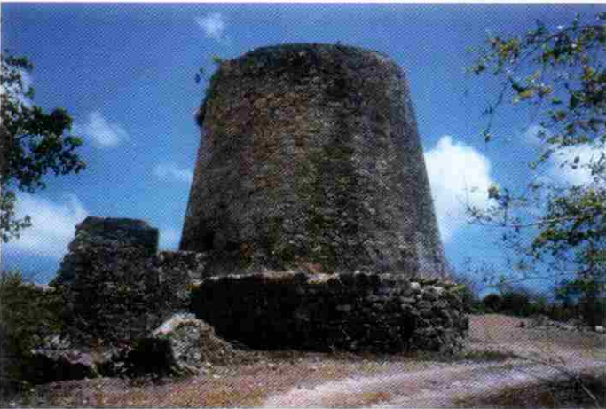
Windmill ruin at Habitation La Mahaudière.
