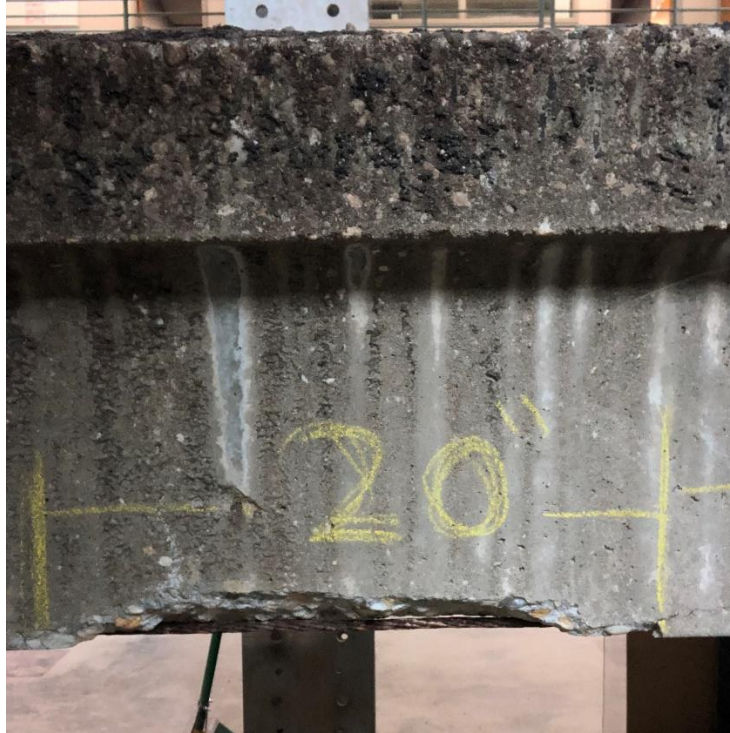
Figure A.36 C10 (NBI 2) moderate defect near midspan.
