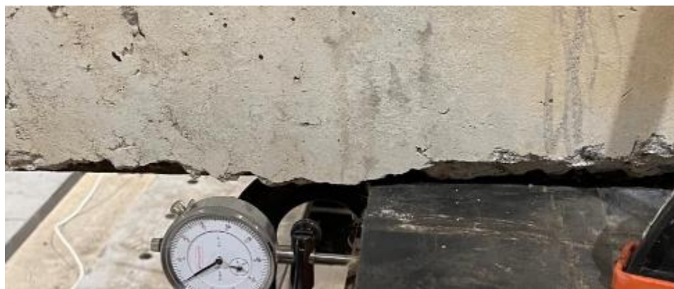
Figure A.17 C5 (NBI 3) major defect.
