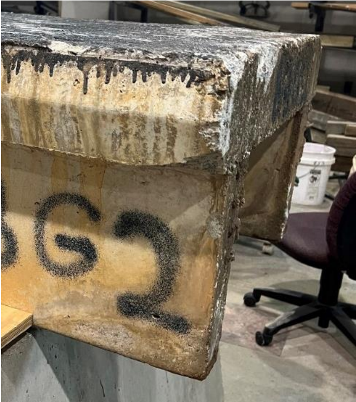
Figure A.51 C12 (NBI 4) end spalling.
