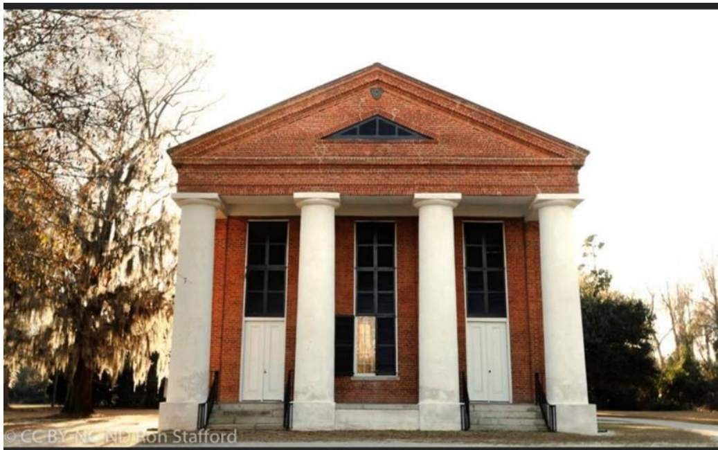
Figure B.1: Front elevation of the Salem Black River Presbyterian Church depicting four columns, two side doors, and a center window. Note the red brick, a unique feature for South Carolina Churches during the nineteenth century.
