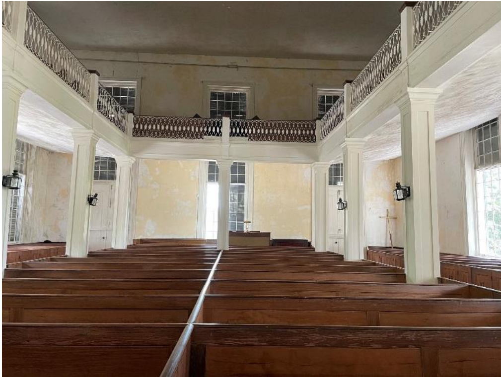
Figure B.2: Interior of Salem Black River Presbyterian. Note the plain walls, windows, and simple floor plan. The Slave gallery extends on three sides and is supported by columns. The Box Pews are also unique to Presbyterian churches, many of which have switched to row pews.
