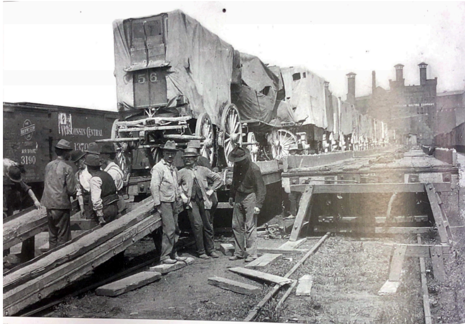
Figure 2.1. Railroad crew unloading circus flatcars using Coup’s “runs” to guide wagons to the ground. Photograph. 1901. Circus World Museum (Reprinted in Dahlinger, Trains of the Circus. )
