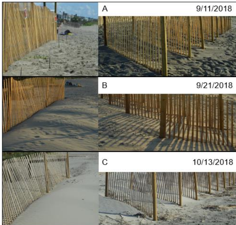
Figure 5.1. Photos of the fenced site on the three collection dates, featuring the shore parallel and oblique fences. A) Pre-Florence; B) Post-Florence/Pre-Michael; C) Post-Michael
