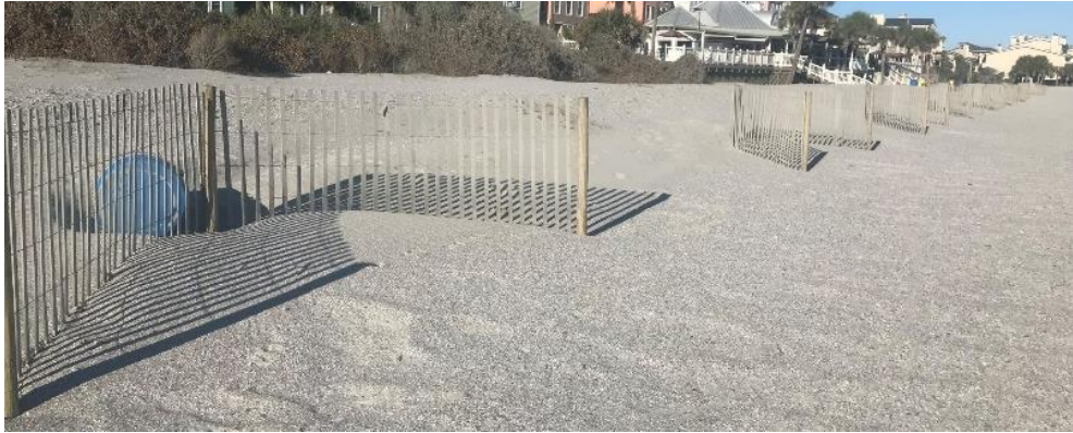
Figure 1.1 Sand fences installed in a V-shaped formation along a South Carolina beach. The apex of the “V” is pointing towards the dune crest.
