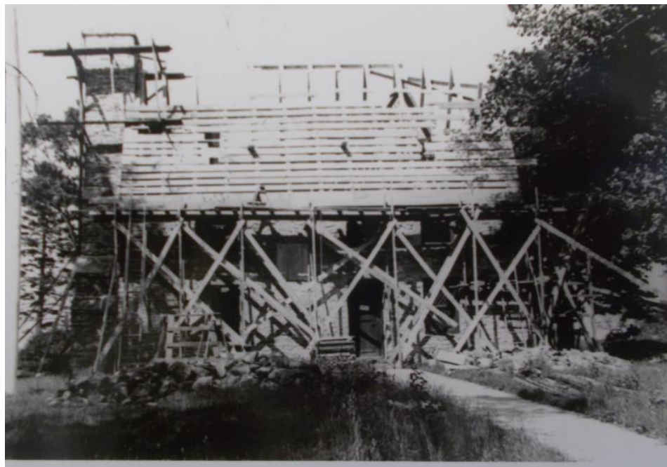
Figure 1.14. WPA workers rebuilding the roof of the Whitfield House. RG 024:001 #3 (top), #52 (bottom), Henry Whitfield House Records, 1768-1957, Photographs, Acc#1958-002, Box 4, Connecticut State Library.
