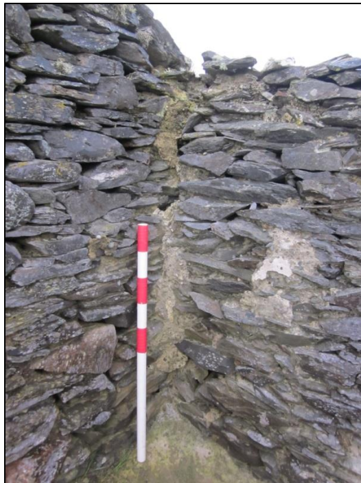
Figure 4.20: Wall abutment with bonded mortar on interior of a house
