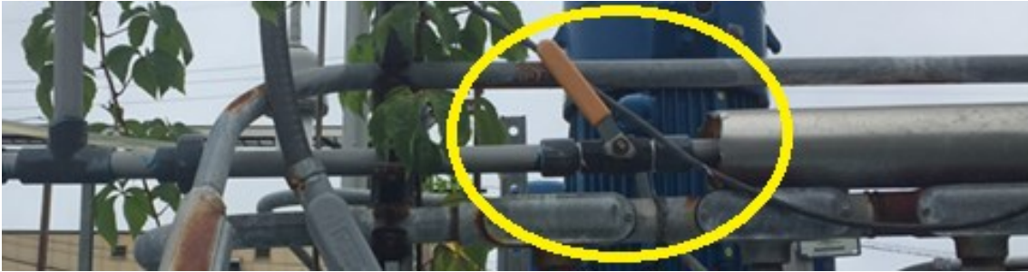
Figure 1.4. Blowdown valve throttled
