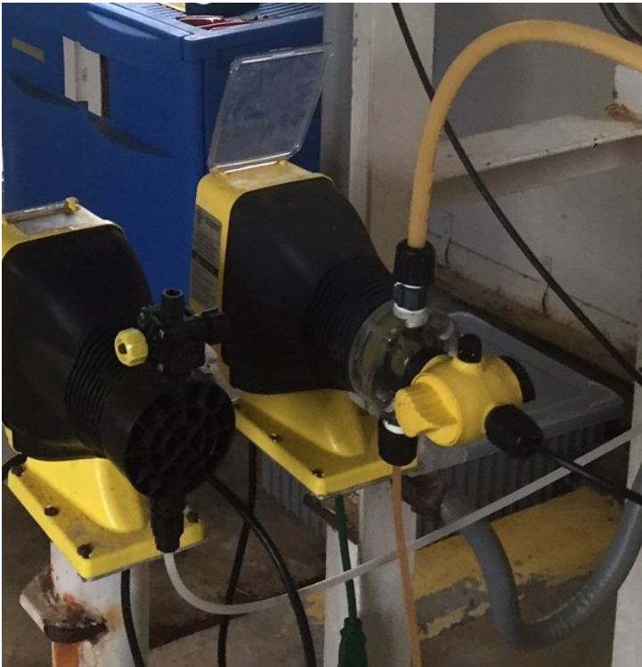
Figure 1.5. CL-49 Metering Pump
