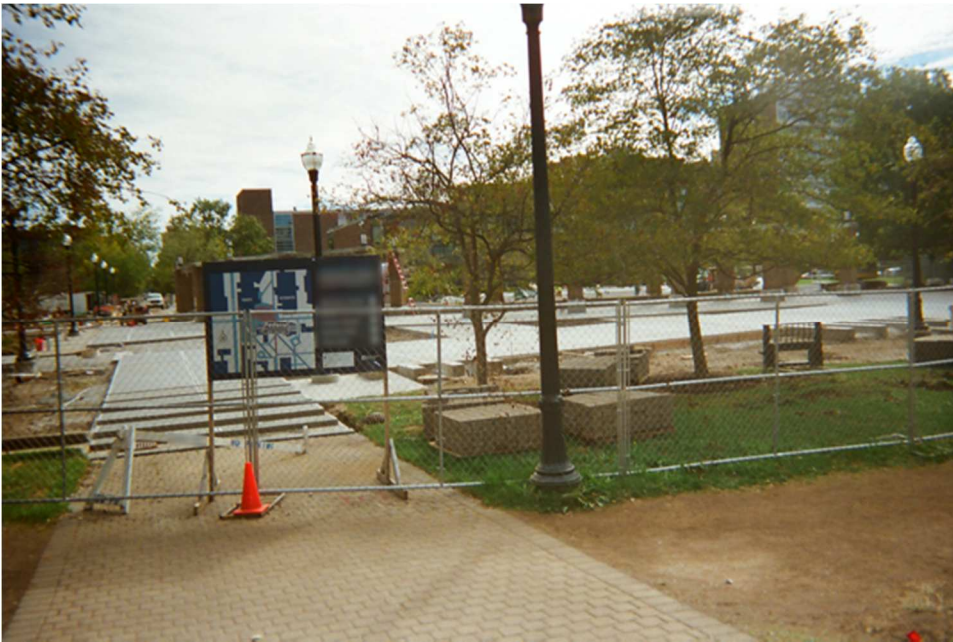
Figure 4.9: Fountain under Construction
