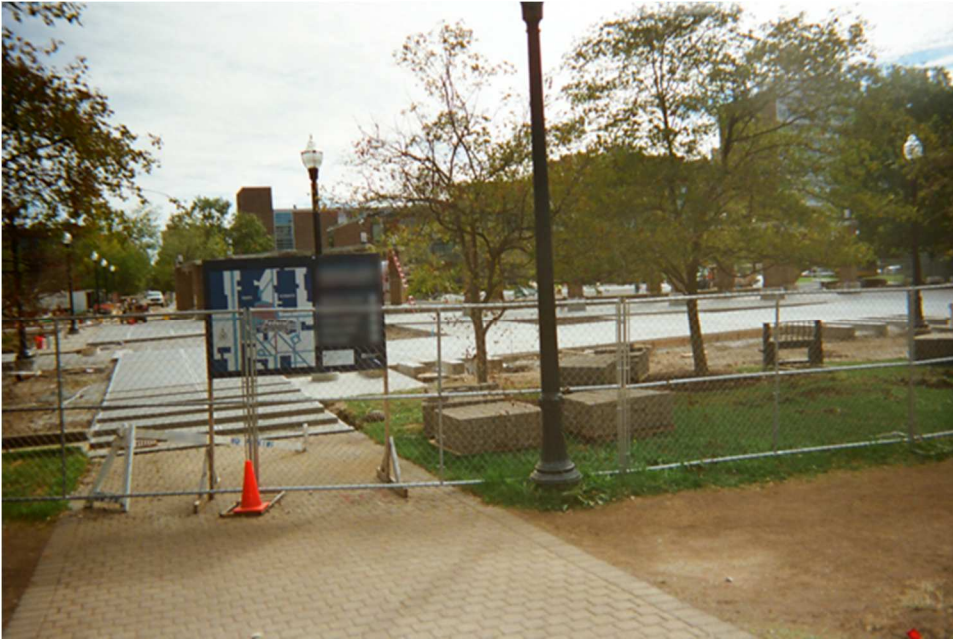
Figure 4.34: Fountain Under Construction
