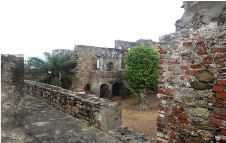
Figure 3.4 Interior view of Fort Amsterdam Portions of walls were demolished during the Dutch-Anglo war, but were rebuilt for tours.
