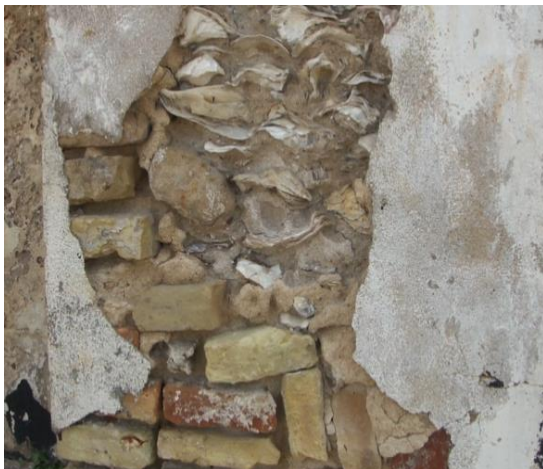
Figure 4.2 Fort Keta's Wall
