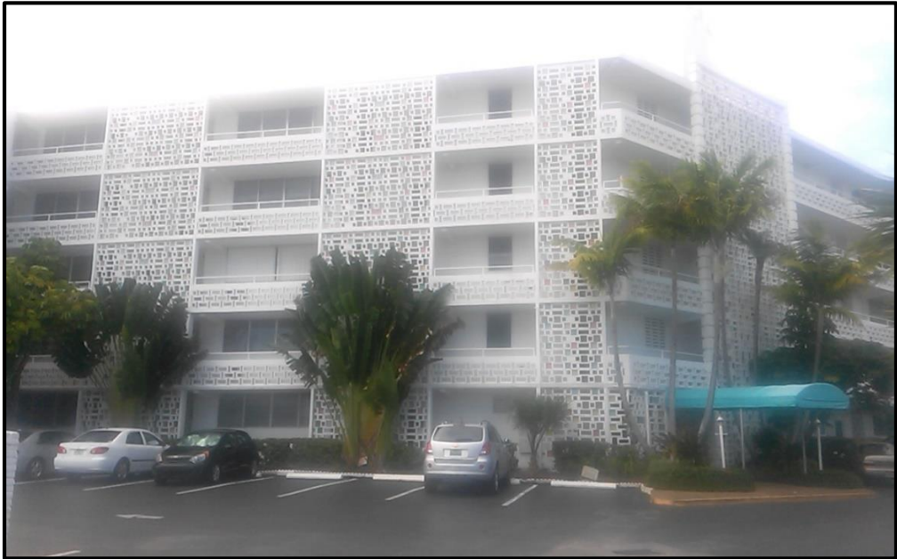
Figure 2.2: Bay Harbor Continental condominium at 1135 103 rd Street. In 2010, the Miami-Dade County Office of Historic Preservation attempted to designate this building as an individual resource. Photographed by author.
