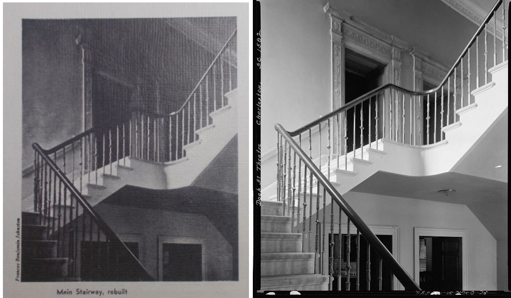
Figure 3.5: Replica staircase in Dock Street Theatre's lobby. Original caption of photography on left: "Central feature of the Lobby is the stairway, a painstaking ferroconcrete replica of the original; since the railing was missing, the architects copied a cast-iron and mahogany contemporary. The magnificent Adam doorways on the landing, leading into the second-floor boxes are originals from the Mitchell King mansion, built in 1805."
