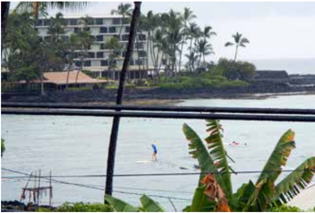
Fig. 7: The 1960's Keauhou Beach Hotel, soon to be demolished, temporarily dominates the NRHP site of Keahou at Kahalu'u Bay; a Heiau platform is at right near the shore. (Photo by Christopher Gillam)
