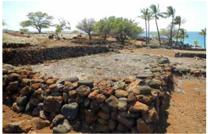
Fig. 3: Dry-stone construction using basalt boulders provided the foundation of traditional Hawaiian architecture, the house wall foundations at Lapakahi State Park. (Photo by Christopher Gillam)
