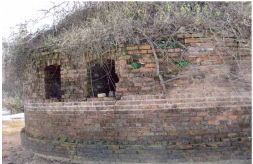
Fig. 1: Brick structure at Ferguson Mill in dry lake bed of Lake Marion. (Photo courtesy of Jim Welch)
