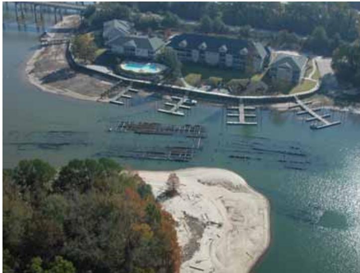
Fig. 3: Several construction barges that were simply left after the dam on Lake Marion was constructed. (Photo courtesy of John C. Dulude, P. E. Manager FERC Relicensing, Santee Cooper)
