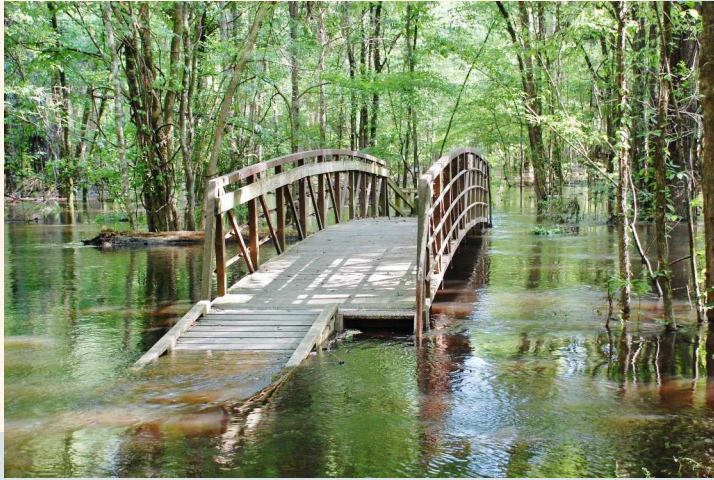
Annual flooding of Cedar Creek
