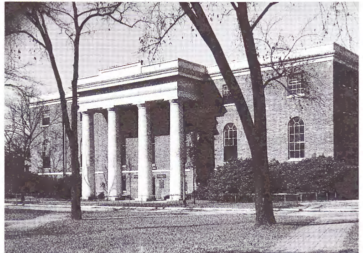
South Caroliniana Library after the addition of the two fireproof wings. Photo from collections of the University Archives.
