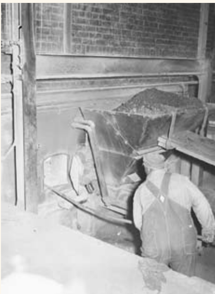
Coal-heating plant, 1940s
