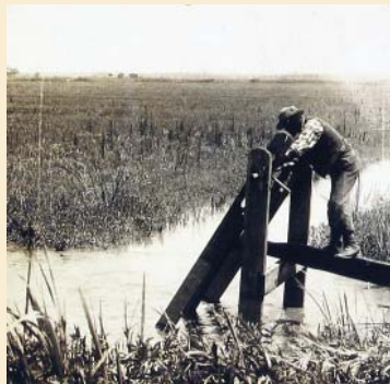
Opening the flood gate
