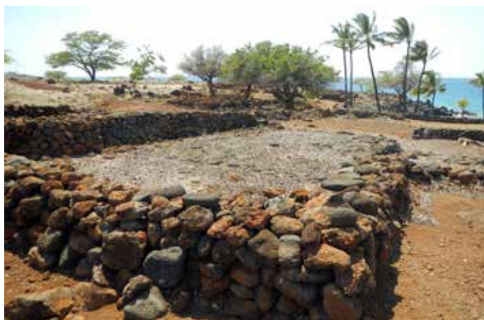
Fig. 3: Dry-stone construction using basalt boulders provided the foundation of traditional Hawaiian architecture, the house wall foundations at Lapakahi State Park. (Photo by Christopher Gillam)
