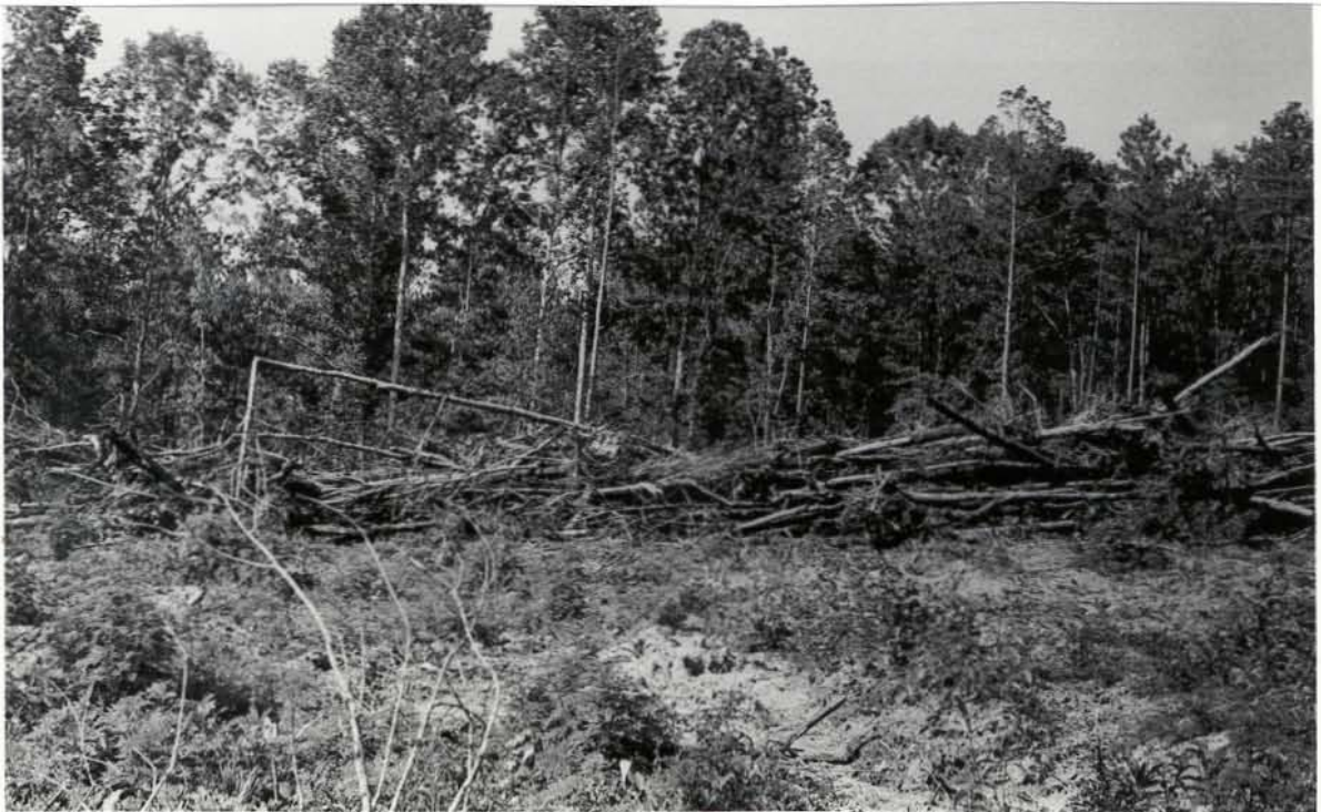
FIGURE 7: A clear-cut area along bridge relocation 2-4. 9EB424 covers slope of hill in the right of the picture.
