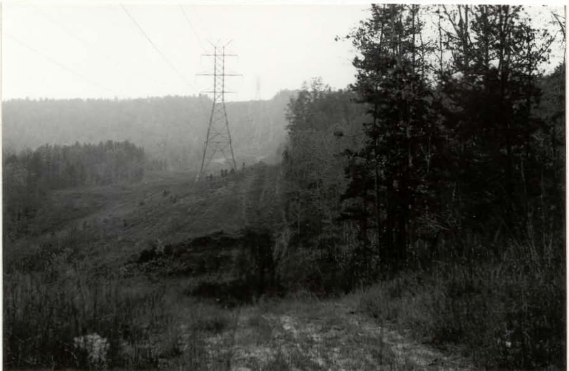
FIGURE 4. Existing 230kv Oconee-Jocassee transmission line corridor in lower part of project area. Vegetation clearing and tower construction may have substantial impact on fragile, close-to-the-surface archeological sites. Corridor will be extended to the right to allow construction of parallel 500kv Oconee-Bad Creek Transmission Line.
