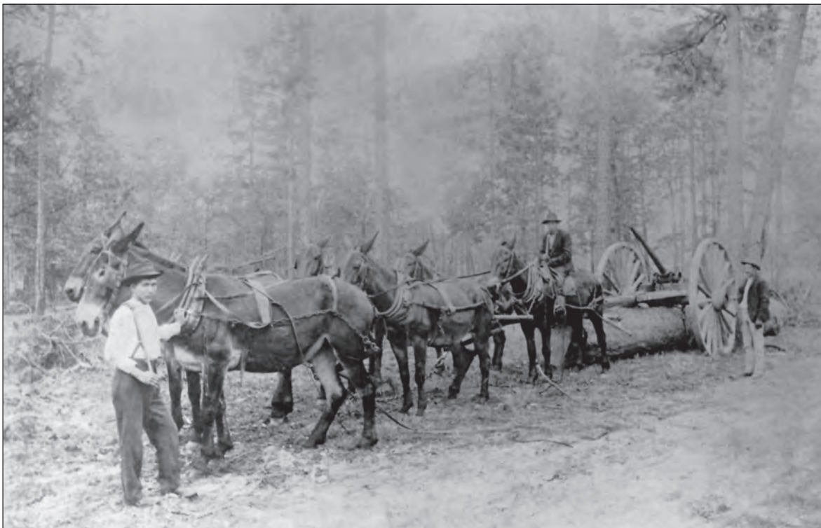
Figure 22 — Early loggers relied on mules and slip-tongue carts to move logs to rivers and mills (courtesy Museum of West Louisiana).
