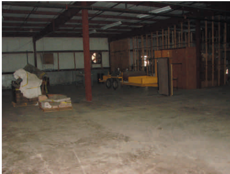
New space for the Curation Facility prior to renovation with new HVAC. When completed, the facility will meet Federal Standards. (SCIAA photo)
