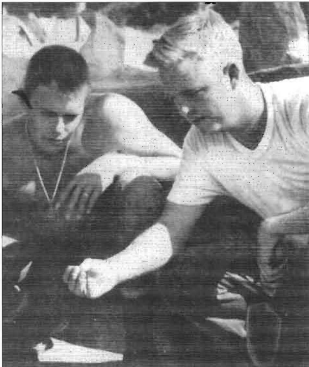
Lewis Binford and Stan South shown here in a photo which appeared in Newsweek , July 4, 1955 (page 76). Digging a feature on the bank of the Roanoke River, they uncovered a hearth feature that dated to 8,000 years ago. (Photo by Sebastian Sommer)
